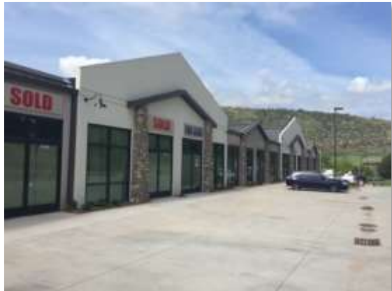
Located at 11616 Shaffer Place in the Ken Caryl Business Center
